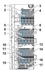
Figure 11. 93PS UPS 30-40 kW power cable terminals
